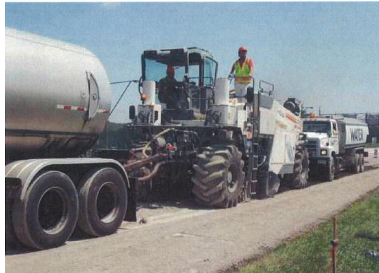
Stabilized Base vs. Unstabilized Base
