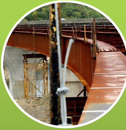
Accelerated Bridge Construction
